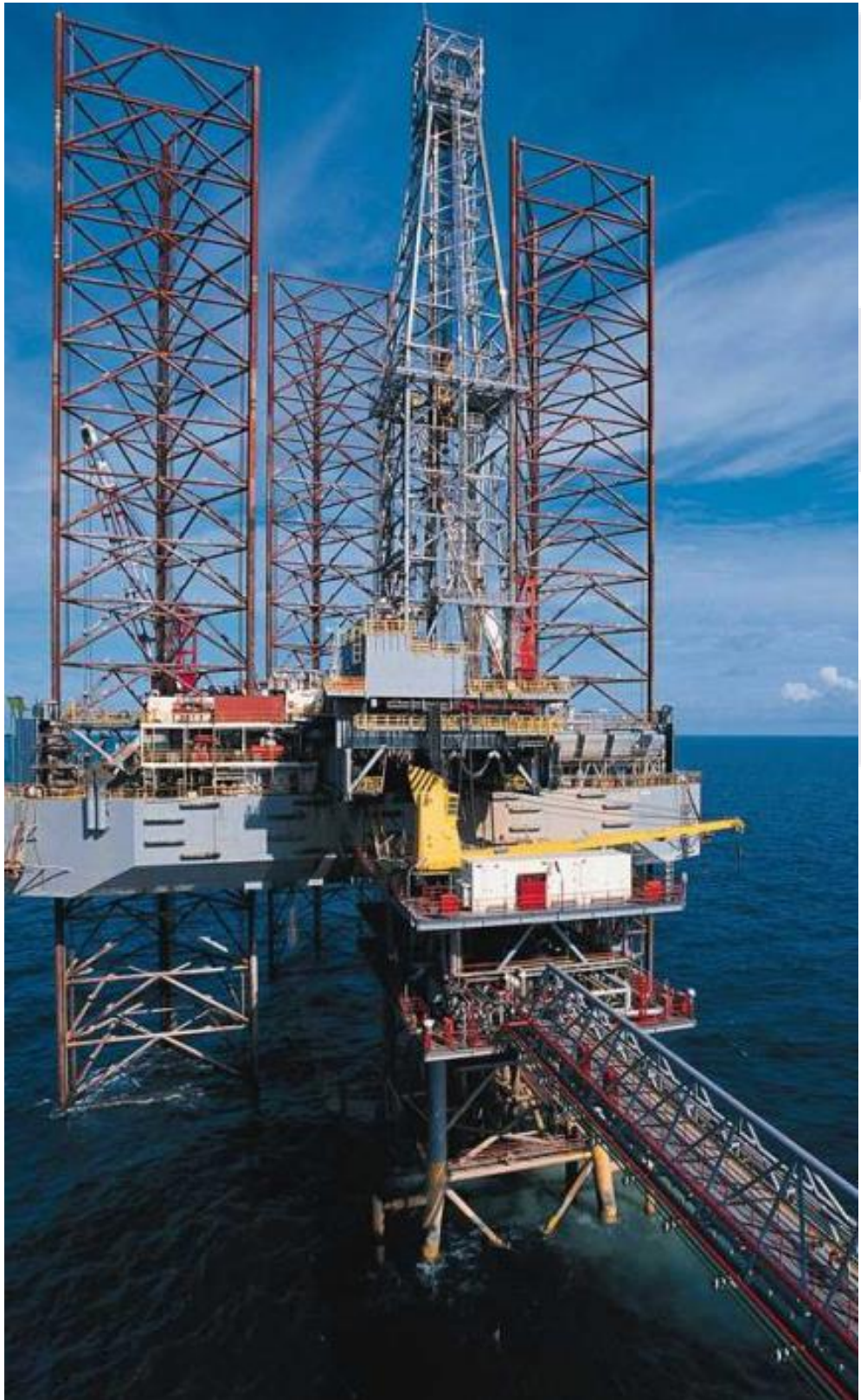
Jack-Up Krathong (Helicopter refuelling system) "Lamprell Energy"
