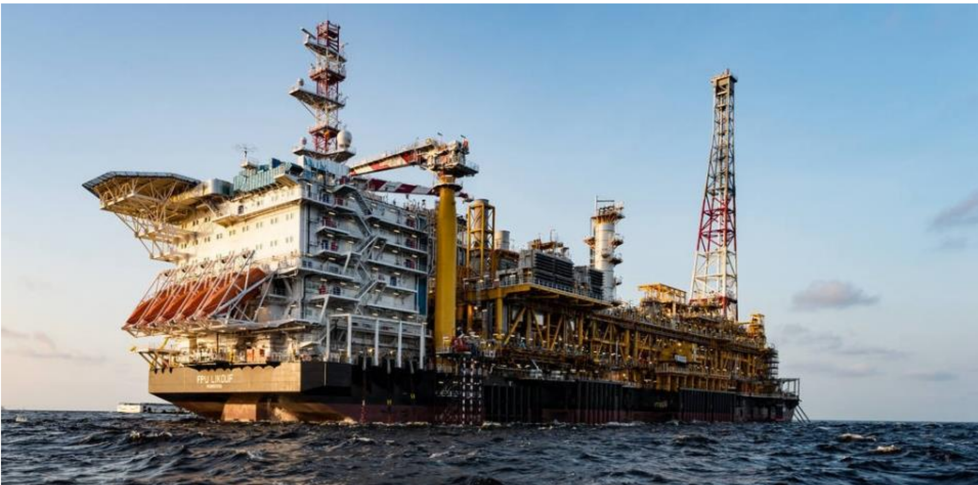
Oily water separator ATEX for TOTAL MOHO FPSO "Hyundai HI"
