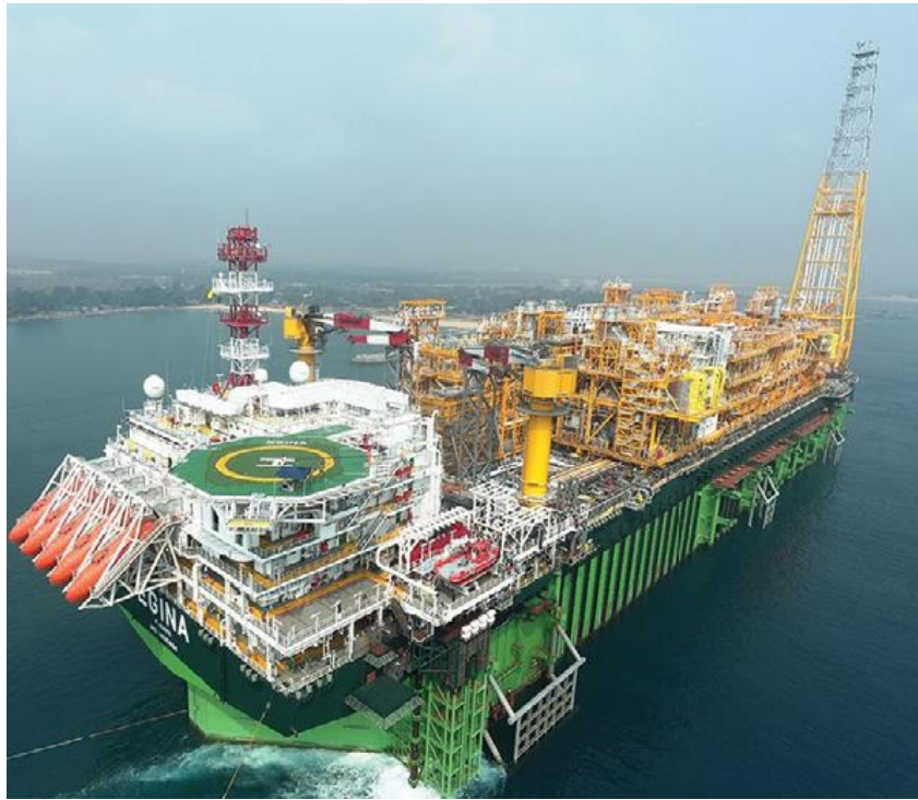
Oily water separator ATEX for TOTAL Offshore Egina FPSO "Samsung HI"
